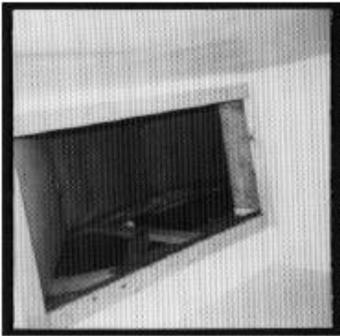
(7) REFRAMED JOIST & ACCESS HOLE
