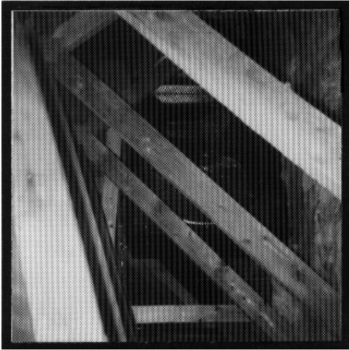
(9) ATTIC VIEW - FRONT LEFT
