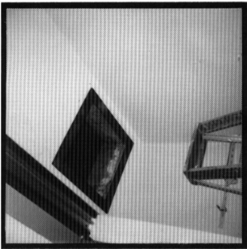
(1) 2X2' EXISTING ATTIC ACCESS
