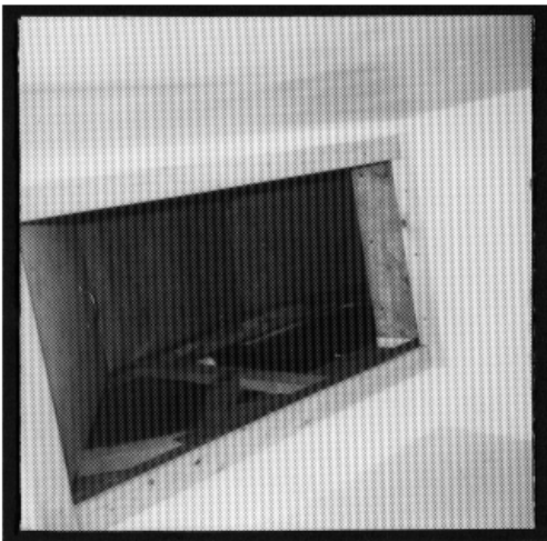
(7) REFRAMED JOIST & ACCESS HOLE
